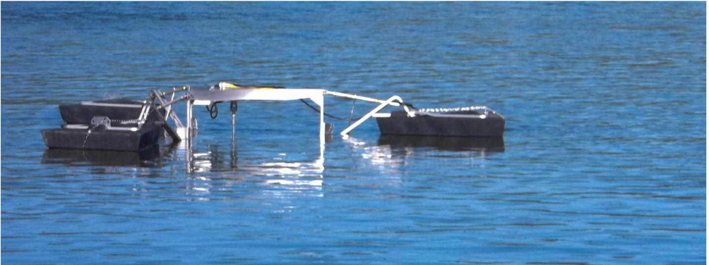
Floating wastewater mixers are a proven odor control strategy for many types of wastewater ponds and basins.
