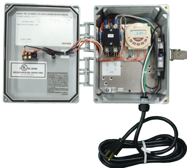
Figure 2: GridBee Timer Disconnect Box, Internal
