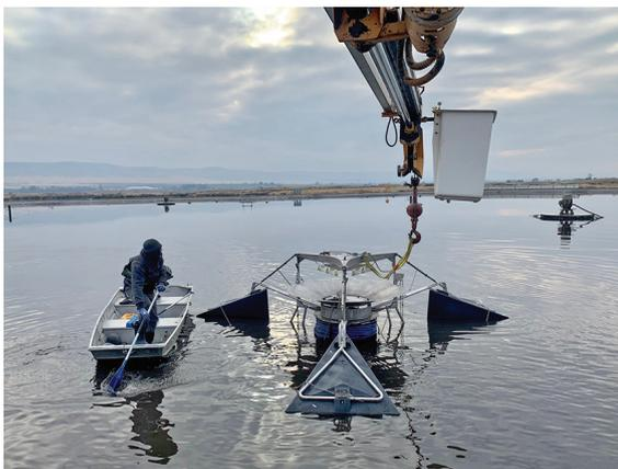
One of four SolarBee mixers being installed using a crane at the Grandview lagoon.
