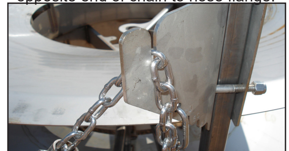
Marker chain slipped into chain bracket slot.
