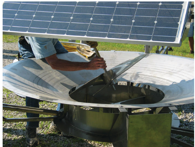
Impeller Removal For Buildup Below Impeller
