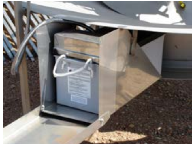
Battery Lid Down, Battery Lead Out
