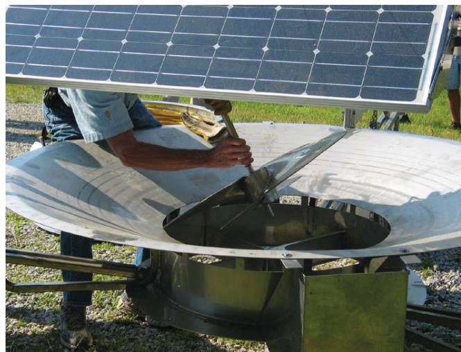
Impeller Removal For Buildup Below Impeller
