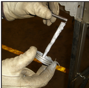
Applying Anti-Seize To The Bolts
