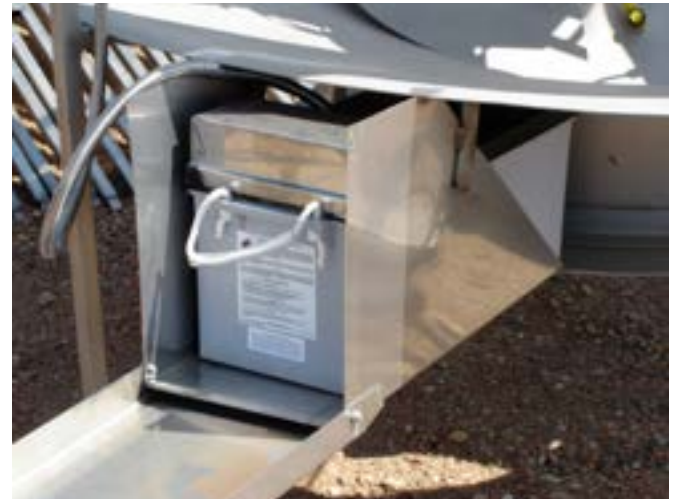
Battery Lid Down, Battery Lead Out
