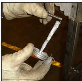
Applying Anti-Seize To The Bolts
