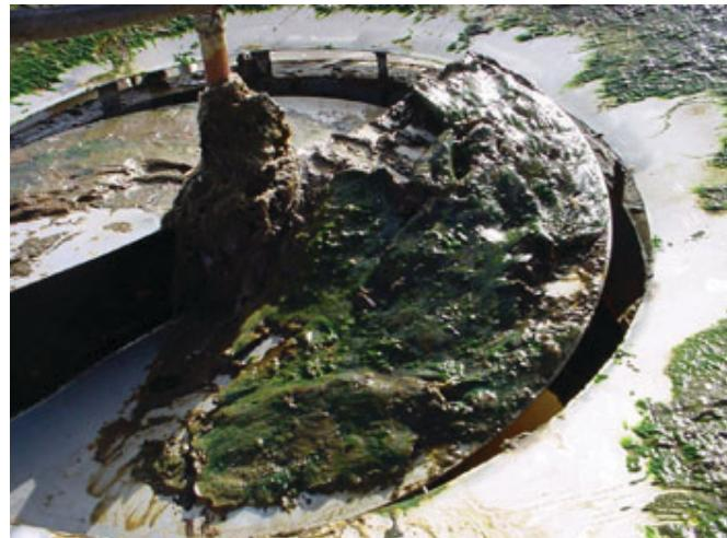
Machine With Buildup On Impeller
