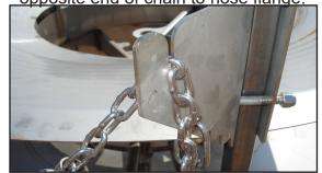
Marker chain slipped into chain bracket slot.
