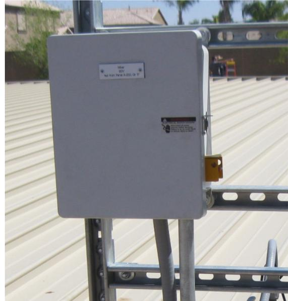
Electronic Control Box of an Underground Reservoir
