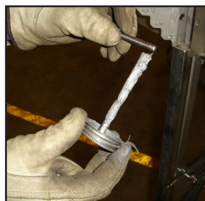
Applying Anti-Seize To The Bolts
