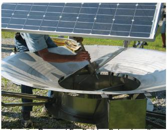
Impeller Removal For Buildup Below Impeller
