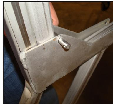
Attaching Leg Extension With a Clevis Pin
