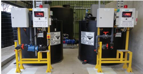
*Ixom Bullet™ self-bunded chemical dosing system (no requirement for expensive concrete bund)*
