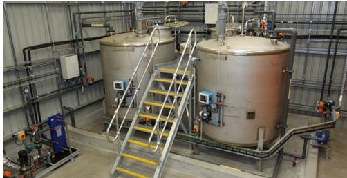
*Contaminated Ground Water Treatment Plant – 60 m<sup>3</sup>/d – Fenton Process – VIC*
