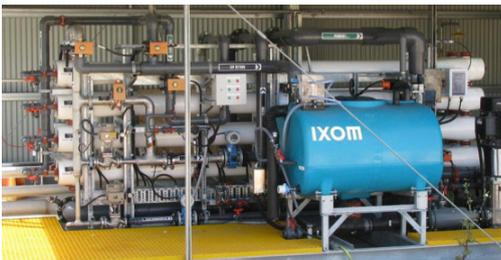
Bore Water Treatment Plant for Boiler Feed Water
