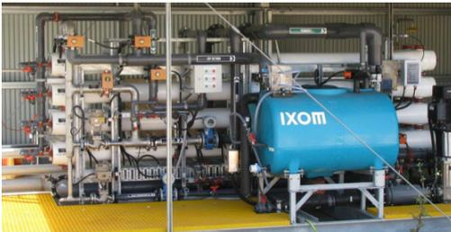
Bore Water Treatment Plant for Boiler Feed Water – 0.9 ML/d – RO – QLD
