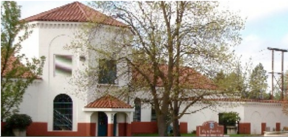
The city's water treatment plant &amp; GridBee® GS-12
