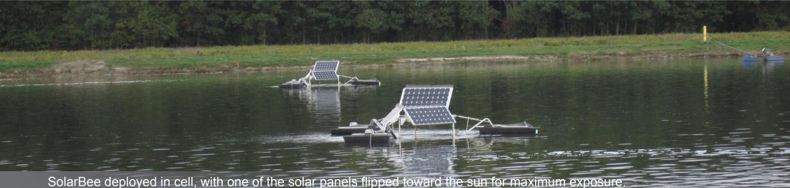
SolarBee deployed in cell, with one of the solar panels flipped toward the sun for maximum exposure.
