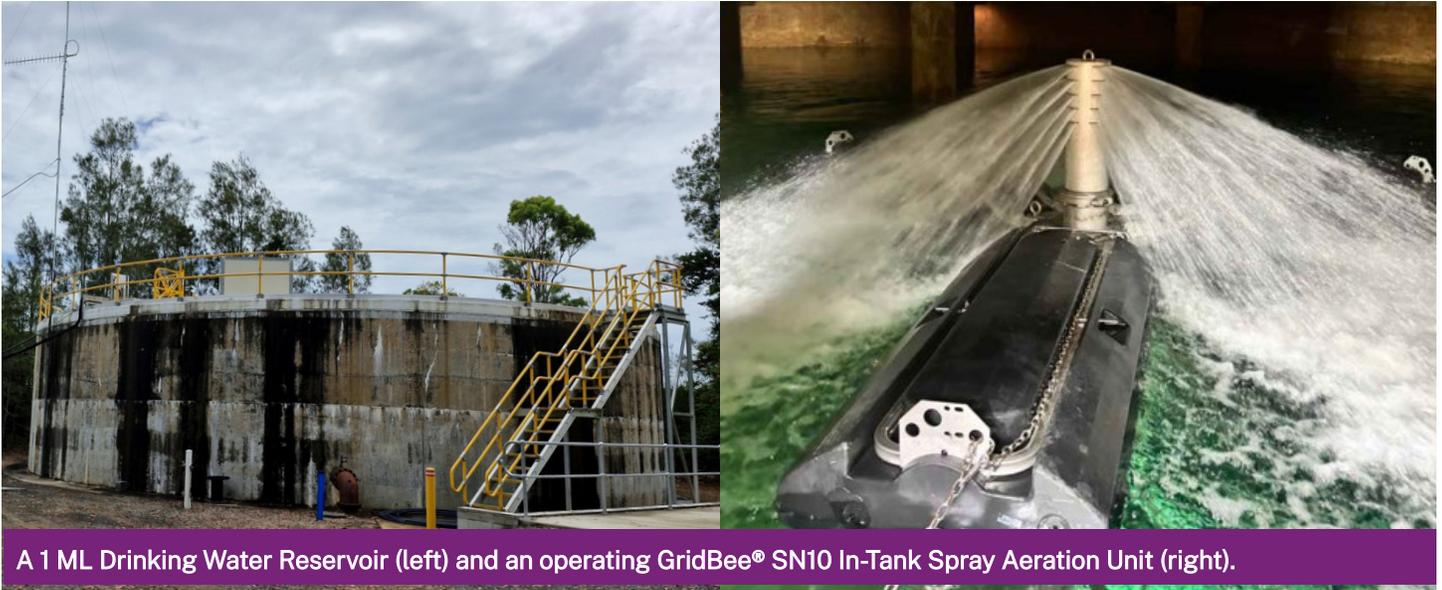
A 1 ML Drinking Water Reservoir (left) and an operating GridBee® SN10 In-Tank Spray Aeration Unit (right).
