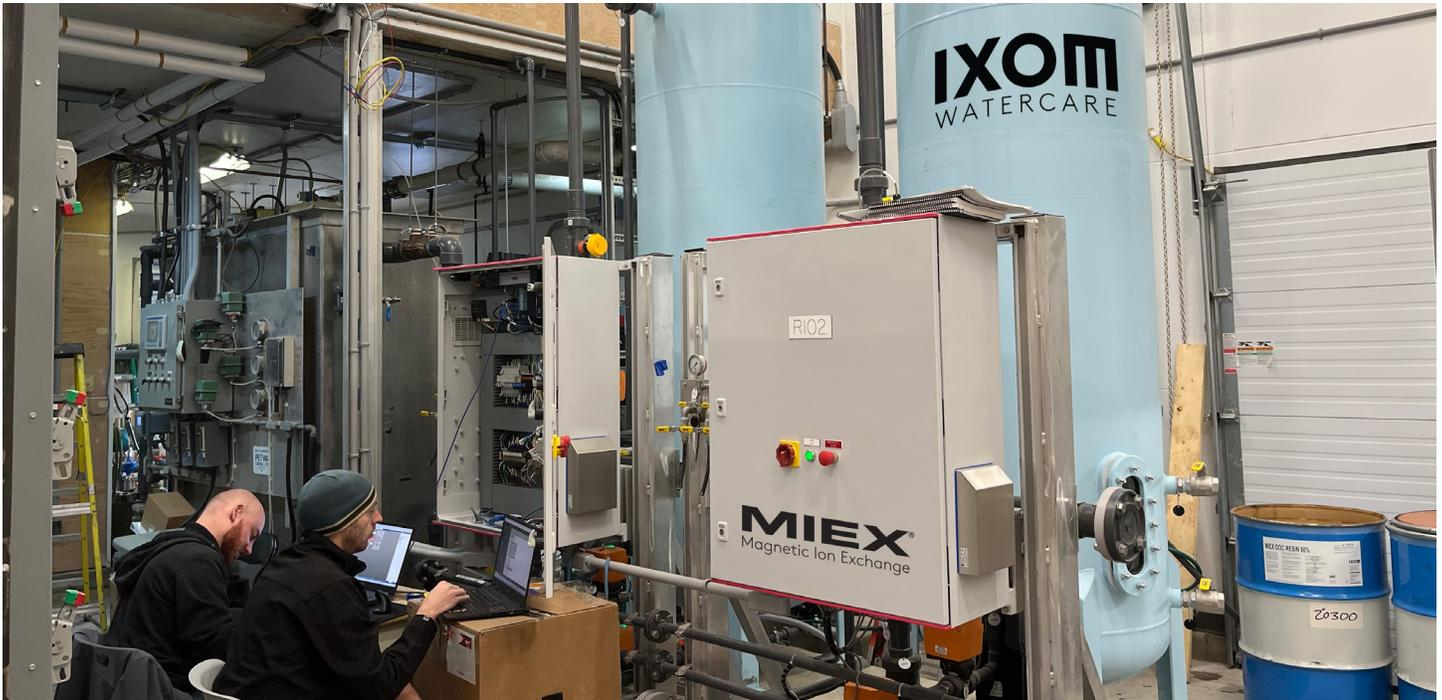
Ixom Watercare Engineers getting the MIEX® Mini Magnetic Ion Exchange System ready to go for initial start-up.
