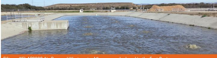
Fifteen (15) AP2000 Air-Powered Wastewater Mixers were deployed in the East Basin.
